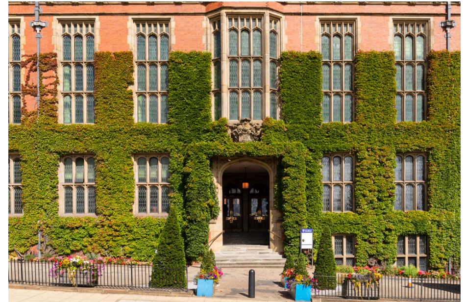
Front entrance to Firth Court. Red brick heritage building with black double doors, large windows and foliage.
